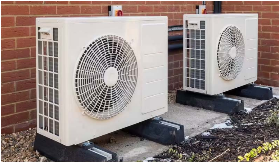
Installation of heating pump
