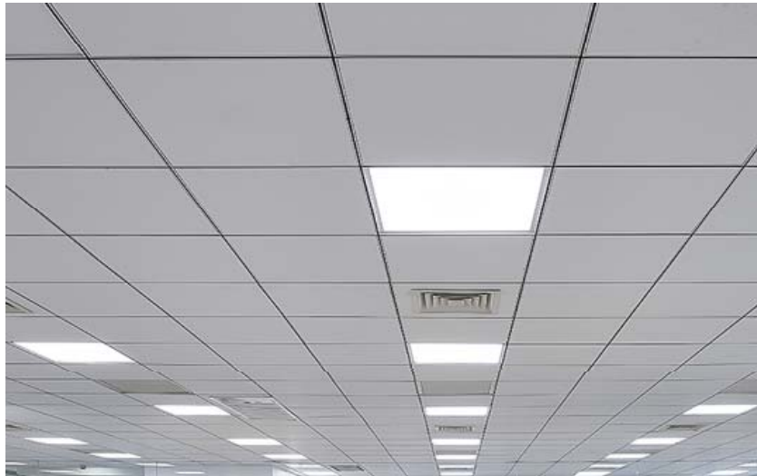
Replacement of the old lighting with new LED technology lighting
